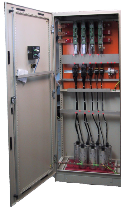
Fig. 3: Switchboard controlled by NOVAR APFC with 7 capacitors
