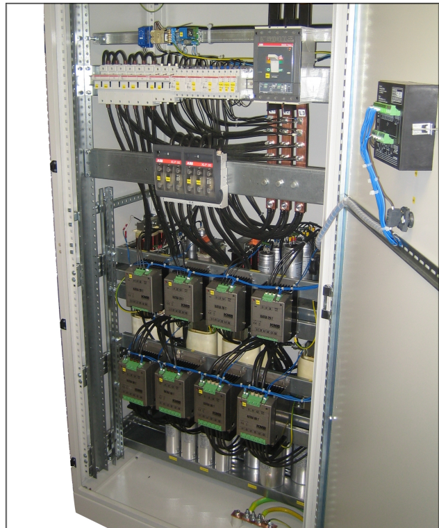
Fig. 2: KATKA thyristor switches controlled by the NOVAR 1312 in fast PFC application
